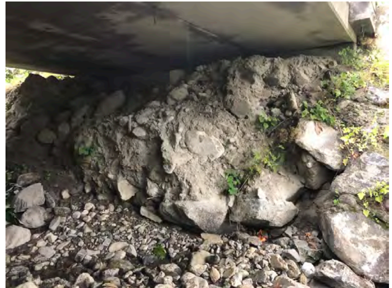
Left Bank Abutment when facing downstream
