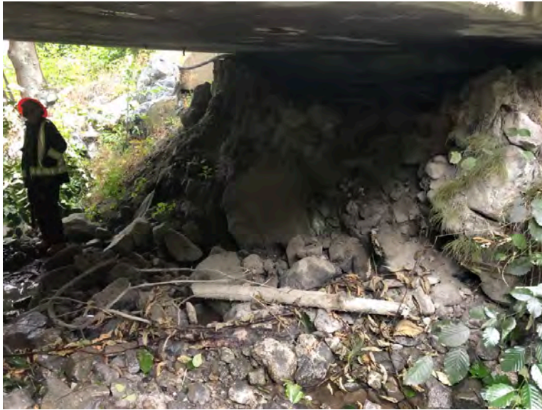
Right Bank Abutment when facing downstream
