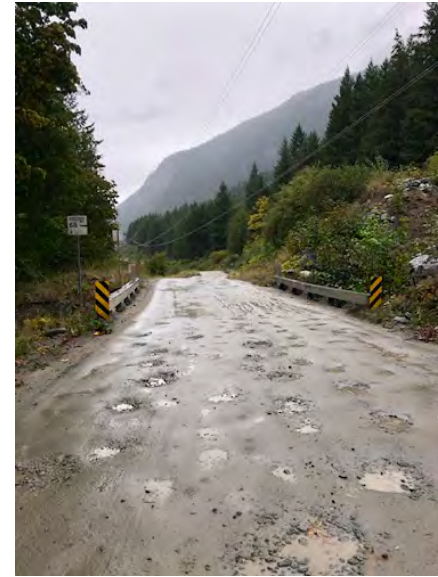
Approach from Right Bank when facing downstream
